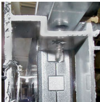
Bohrschrauben Self-drilling screws
